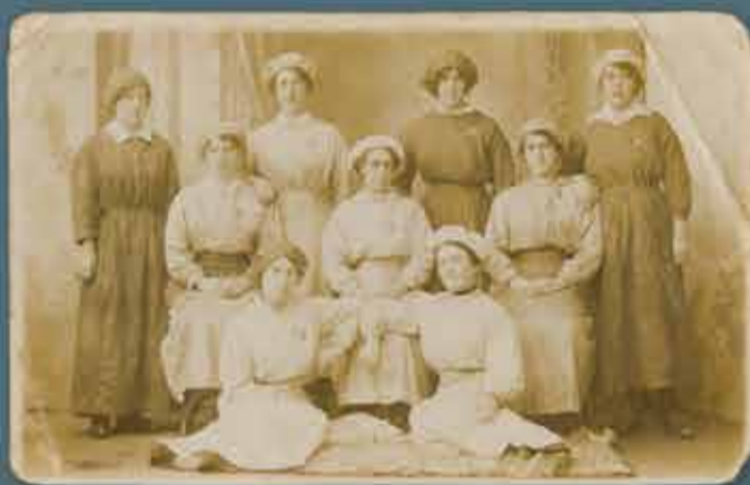
Workers at the Vulcan Munitions Factory, Quarry Bank, Caernarfon . They all have triangular war-workers badges.
